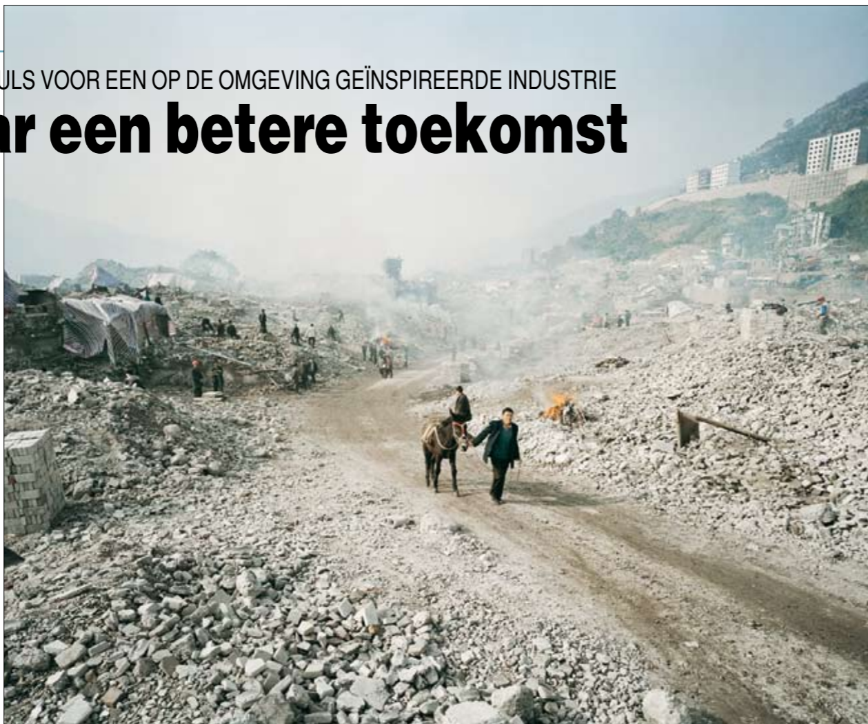
Dam, Three Gorges Dam Project, Yangtze River, 2005 Courtesy Edward Burtynsky, Toronto, Canada
